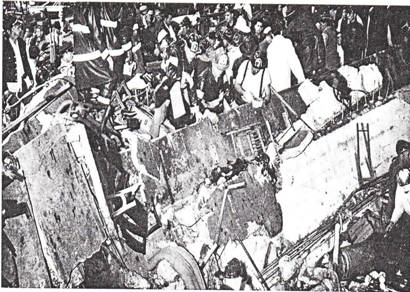
PLATE II—BLAST AREA. Note the size of concrete rubble and the LP gas tank in the lower right hand corner of the picture. Courtesy of The Indianapolis Times .
