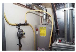
Homeowners and property owners who have yellow CSST installed in their homes are encouraged to determine if the system is properly bonded. Licensed electrical contractors should be contacted to make the correct determination on proper bonding of the system. Costs associated with performing this
