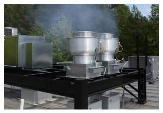
When a hinge kit is installed, a fixed location fan is far more stable and less likely to have problems with balance and bearing misalignment due to limited movement allowed during normal operations and during the inspection and cleaning process. Properly installed hinge kits add to the strength of
