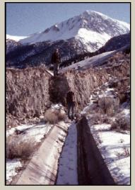
Peak earthquake in Idaho (surface faulting has broken and offset the concretelined ditch in which the people are standing). Over time, repeated movement on a normal fault eventually produces a mountain range on the uplifted crustal block (for example, the Wasatch Range) and a valley or basin on the downdropped block (for example, Salt Lake Valley). (Photo courtesy of Walter Arabasz)
