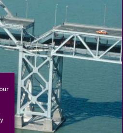
The 1989 magnitude 6.9 Loma Prieta earthquake caused this section of the San Francisco-Oakland Bay Bridge to collapse. (Photo courtesy of USGS)
