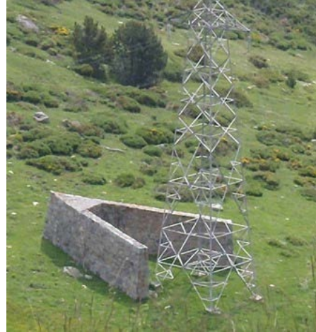
Masonry Deflection Wedge, Val d'Aran, Spain Source Chris Wilbur
