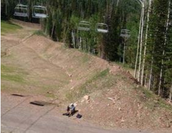
Deflection Dam, Park City, Utah Source Chris Wilbur
