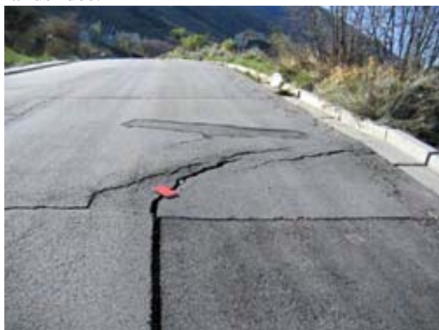
Damage to road in upper part of Sherwood Hills landslide, Provo, courtesy UGS.
